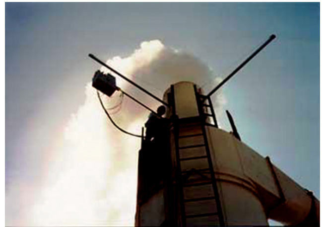
Figure 4: Example of an unsuitable sampling location
