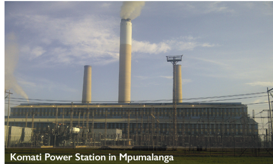
Komati Power Station in Mpumalanga
