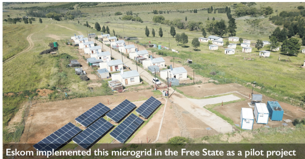
Eskom implemented this microgrid in the Free State as a pilot project
